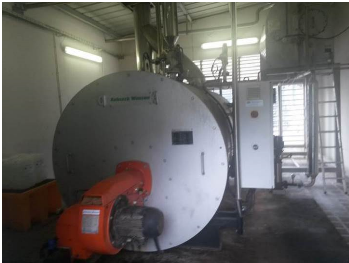
Figure 23 : Chaudière
